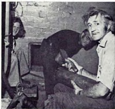
Working on the cables. From left to right: Messrs. David McCann (apprentice electrical fitter), George Johnson (jointer) and Jock Kerr (jointer's mate).
