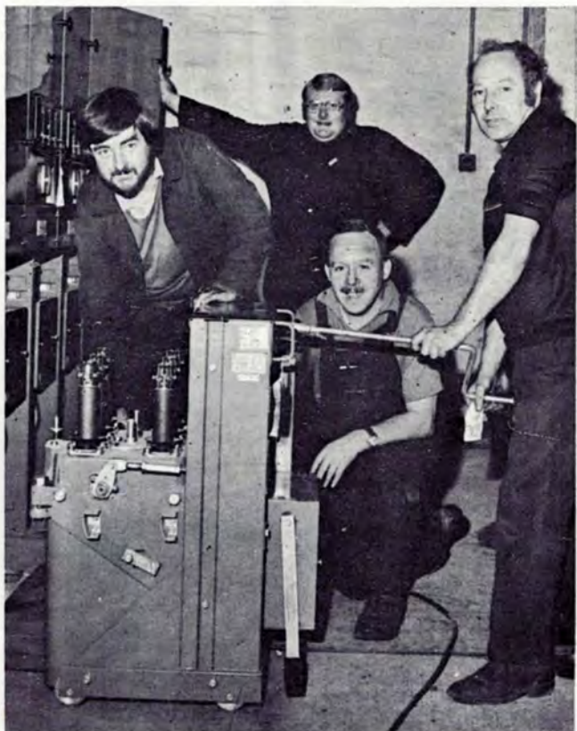
Installing the new switchgear. From left to right: Messrs. Jack Higham (fitter), Dave Harvey (fitter)—holding the board up!— Larry Marr (fitter's mate) and Bill Harris (fitter).
