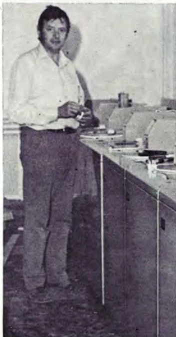
Wiring up the washing machines in the Centre's laundry room is Mr. Raymond Evans (chargehand electrician)
